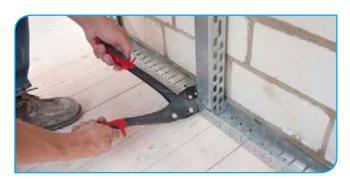
The design ensures that the installation lines for electricity and water can be easily passed through the wall without having to punch the otherwise customary additional passages, as is required with standard studs. The ergonomic and efficient design reduces the working time required, decreasing the cost of labour in construction, which makes MAXI-TEC\* an economical solution for all applicators.
